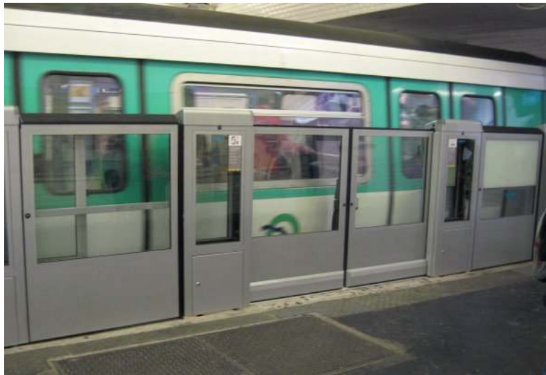
Figure 2. COPPILOT Platform Screen Door
